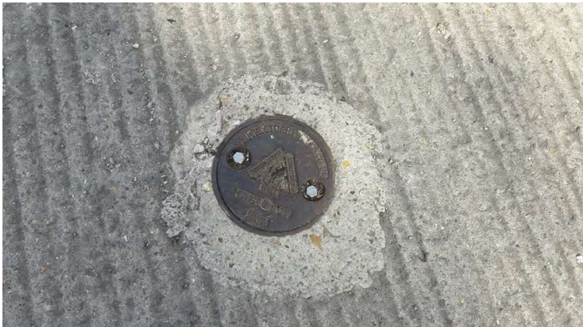
Plate 8: One of four boreholes installed by Leap in 2015
