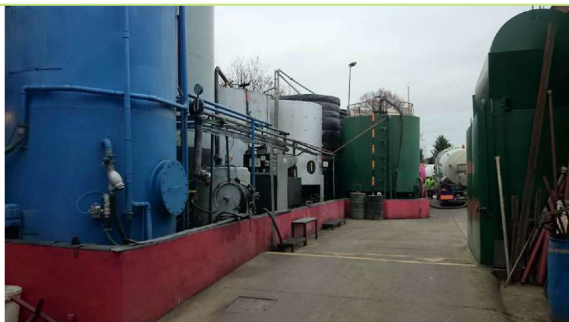
Plate 20 – South end of tank farm
