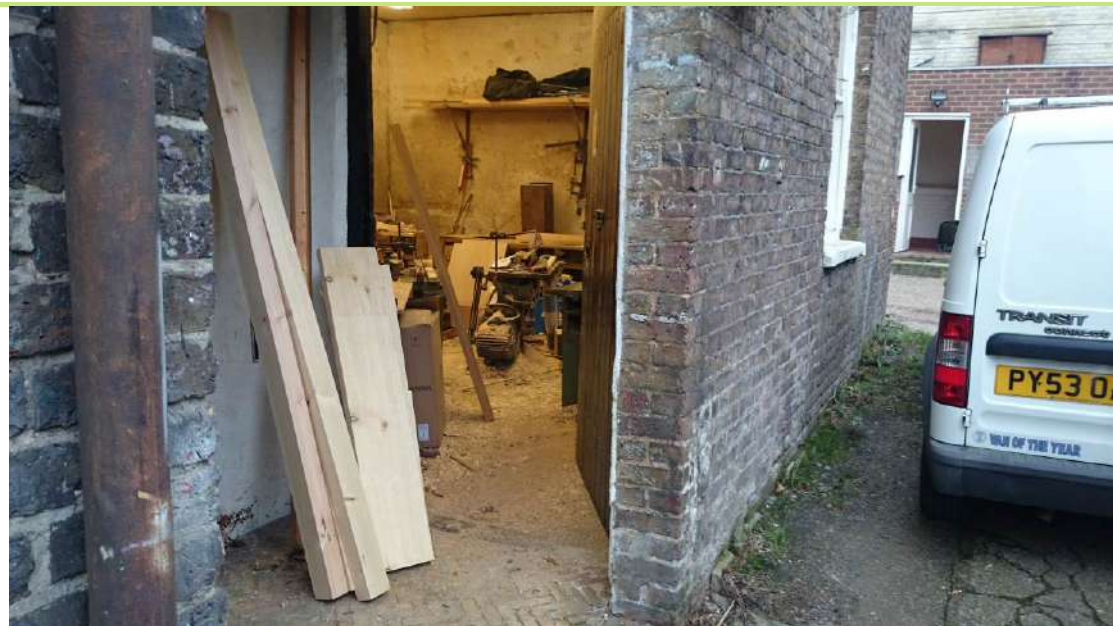
Plate 22 – Joinery workshop within eastern coach house (south end)
