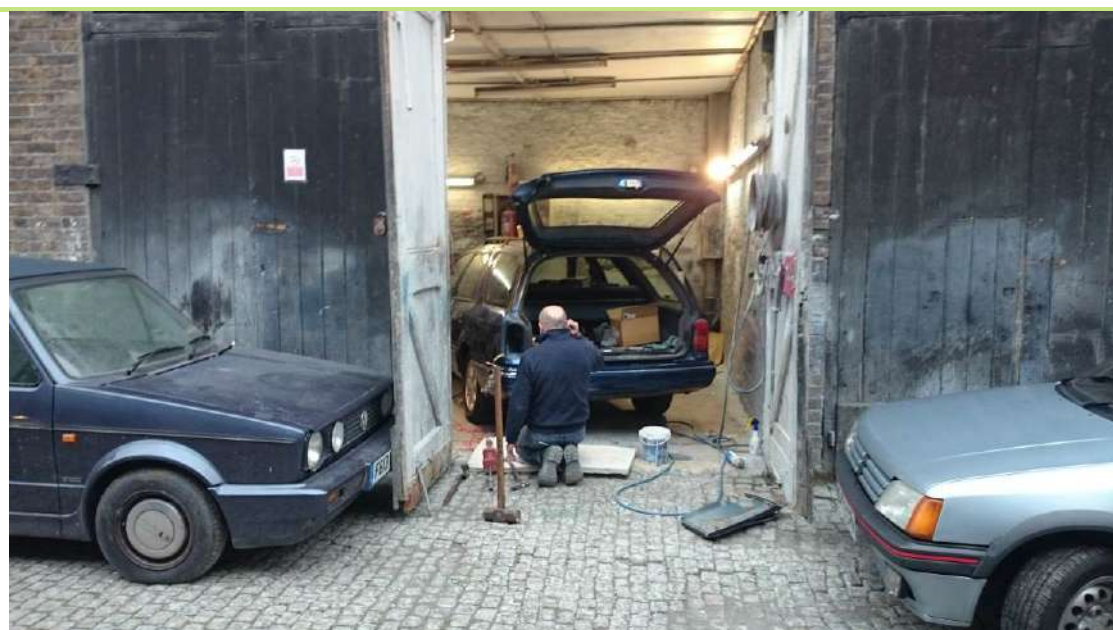
Plate 22 – Car body repairs within western coach house
