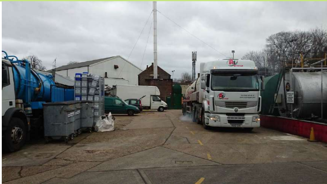
Plate 13 – Tanker loading/unloading alongside tank farm.
