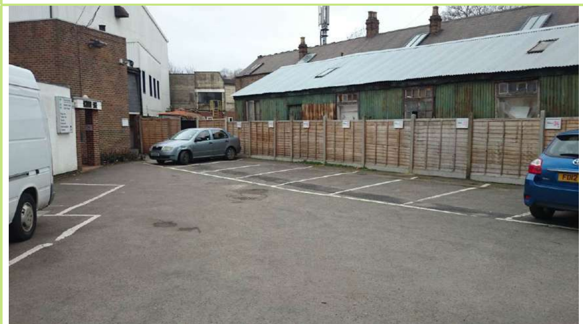
Plate 32 – Studios car park
