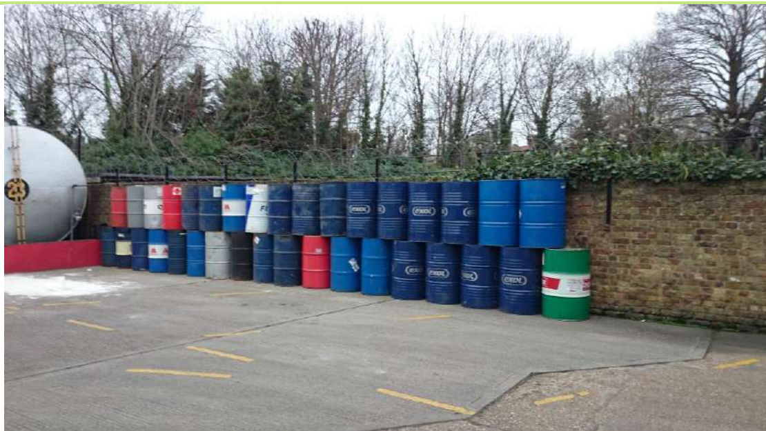
Plate 14 – Barrels along the northern side of drive at northern end of tank farm.
