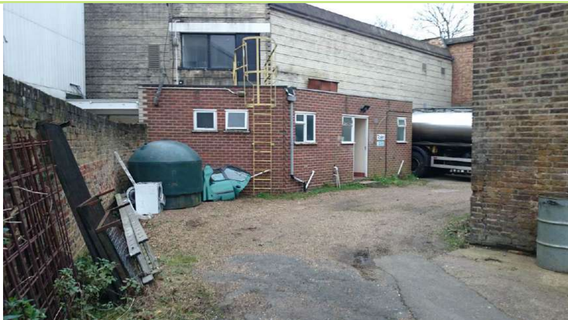
Plate 25 – Toilet building at southwest end of site
