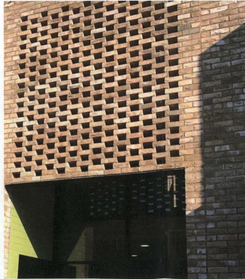
Ely Court by Alison Brooks Architects
