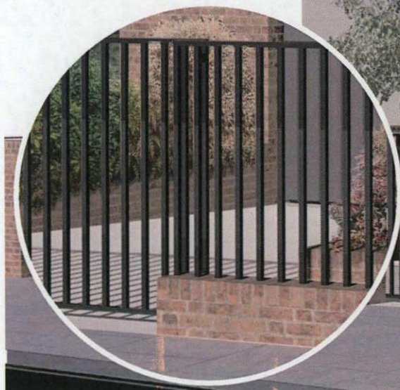
Weinerberger Kenilworth Antique brick or similar at low level with black metal railings above
