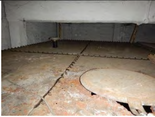
A view of the top of the water tank described above.
