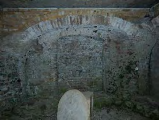
View of the extent of the interior of the grotto, for which brickwork is largely intact, lacking many crevices
