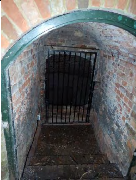
View from ice house exterior door into passageway with grill to sunken ice house in background
