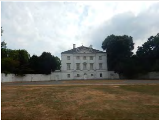
Context of northern elevation
