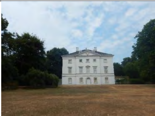
Context of southern elevation
