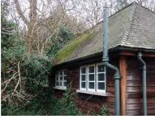
A picture showing the south-west aspects of the coach house store building, with the wooden panelled walls and tiled roofing.
