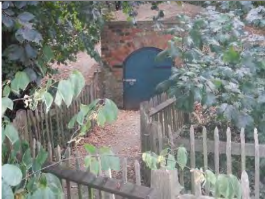
A view of the context of the front of the ice house
