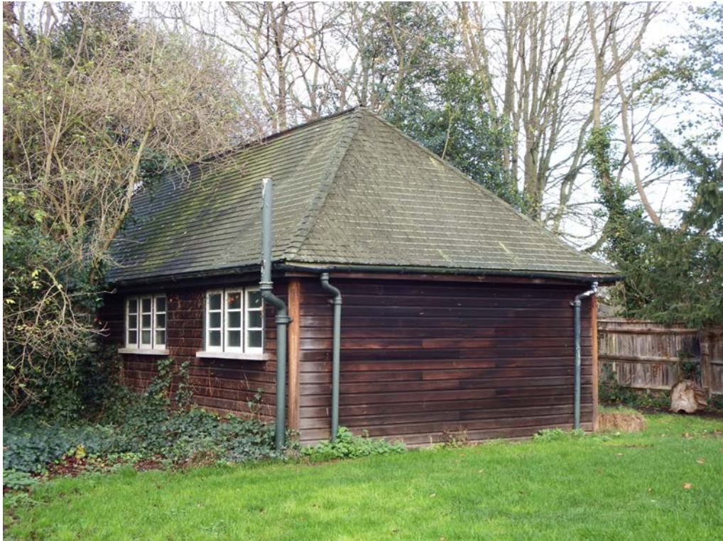
Fig 39 The former dressing rooms, now used for storage
