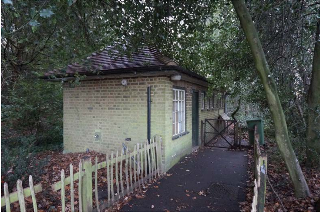
Fig 36 The former ladies' convenience block, now used for storage
