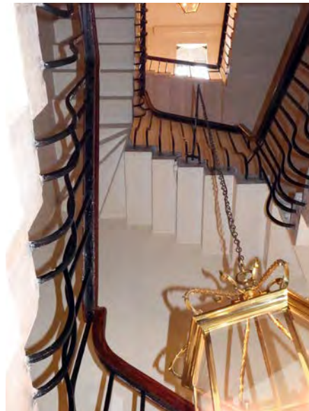
Fig 87 Secondary or service staircase
