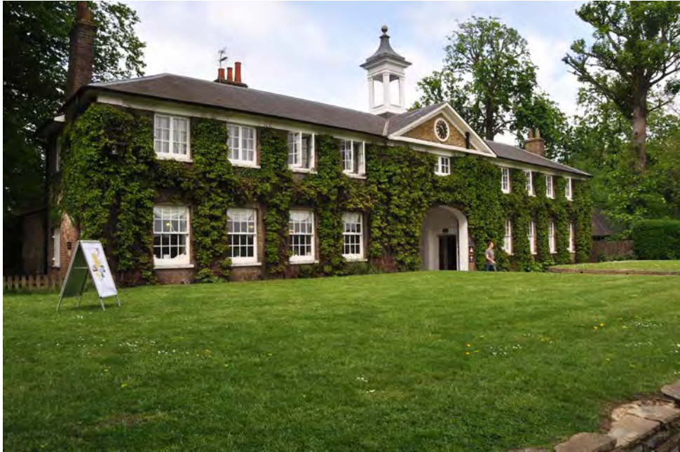
Fig 88 The front of the Stable Block
