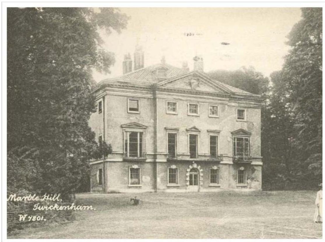
Fig. 5 Marble Hill House, south elevation showing 19 th -century alterations.
