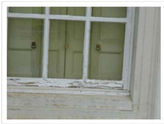
Fig. 16a & 16b Decay of window joinery.
