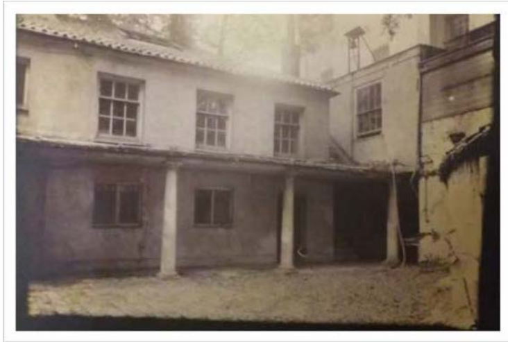
Fig. 4 Marble Hill House service wing (built 1738). View from the sunken courtyard.
