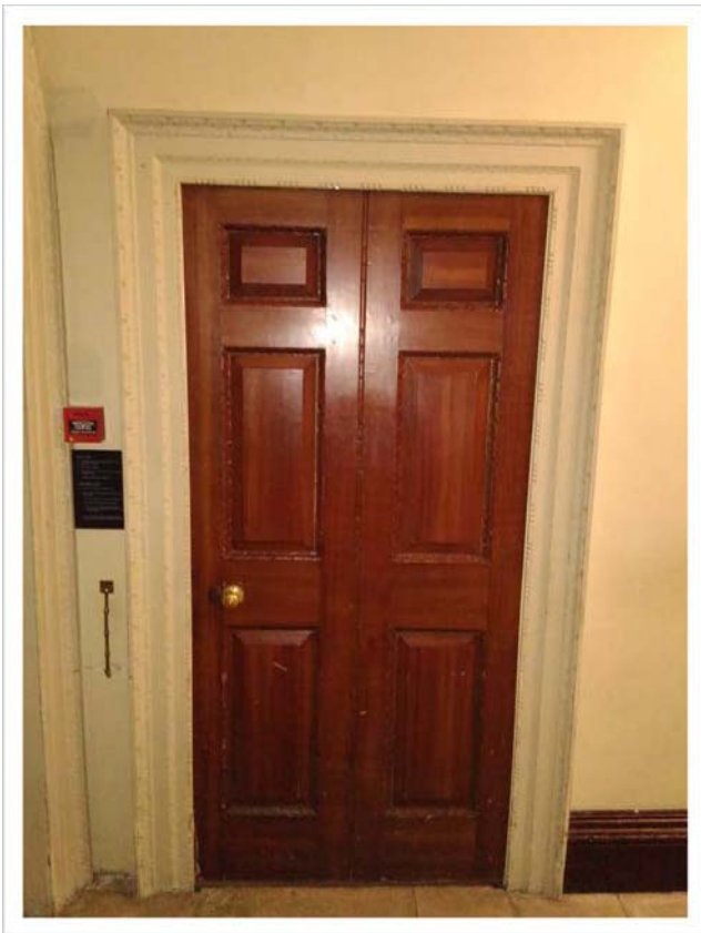
Fig. 10 A typical period-style door to be upgraded with fire retardant sealant and intumescent paint.
