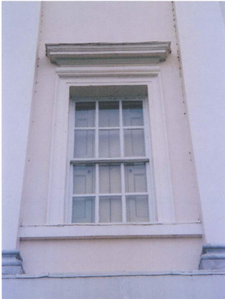
Figure 14). Exterior North façade, detail of the first floor central window
