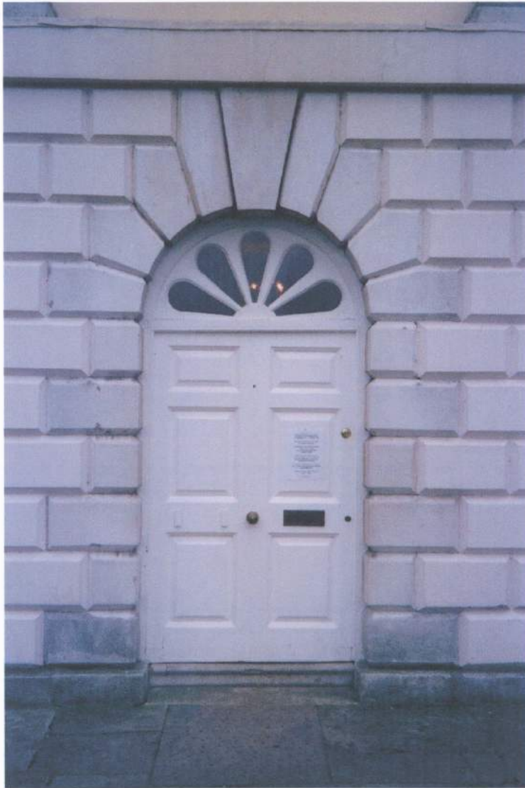
Figure 16). Exterior North façade, Main Entrance Door
