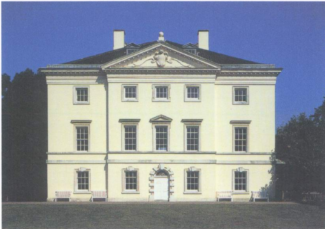
Figure .10). . View of the South façade of Marble Hill House, showing the modern scheme as it appeared in February 2004
