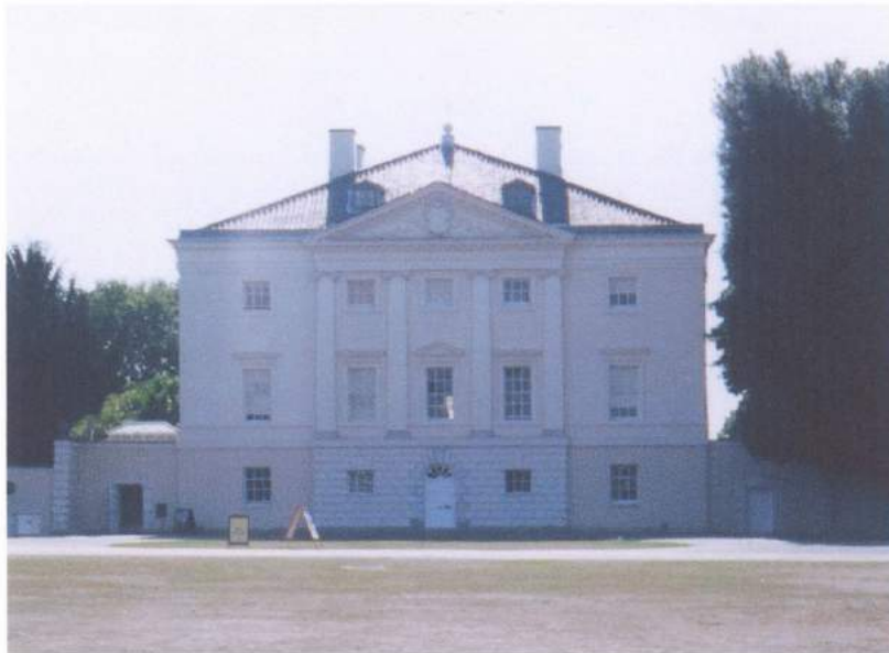
Figure 12). Exterior North façade, September 2003
