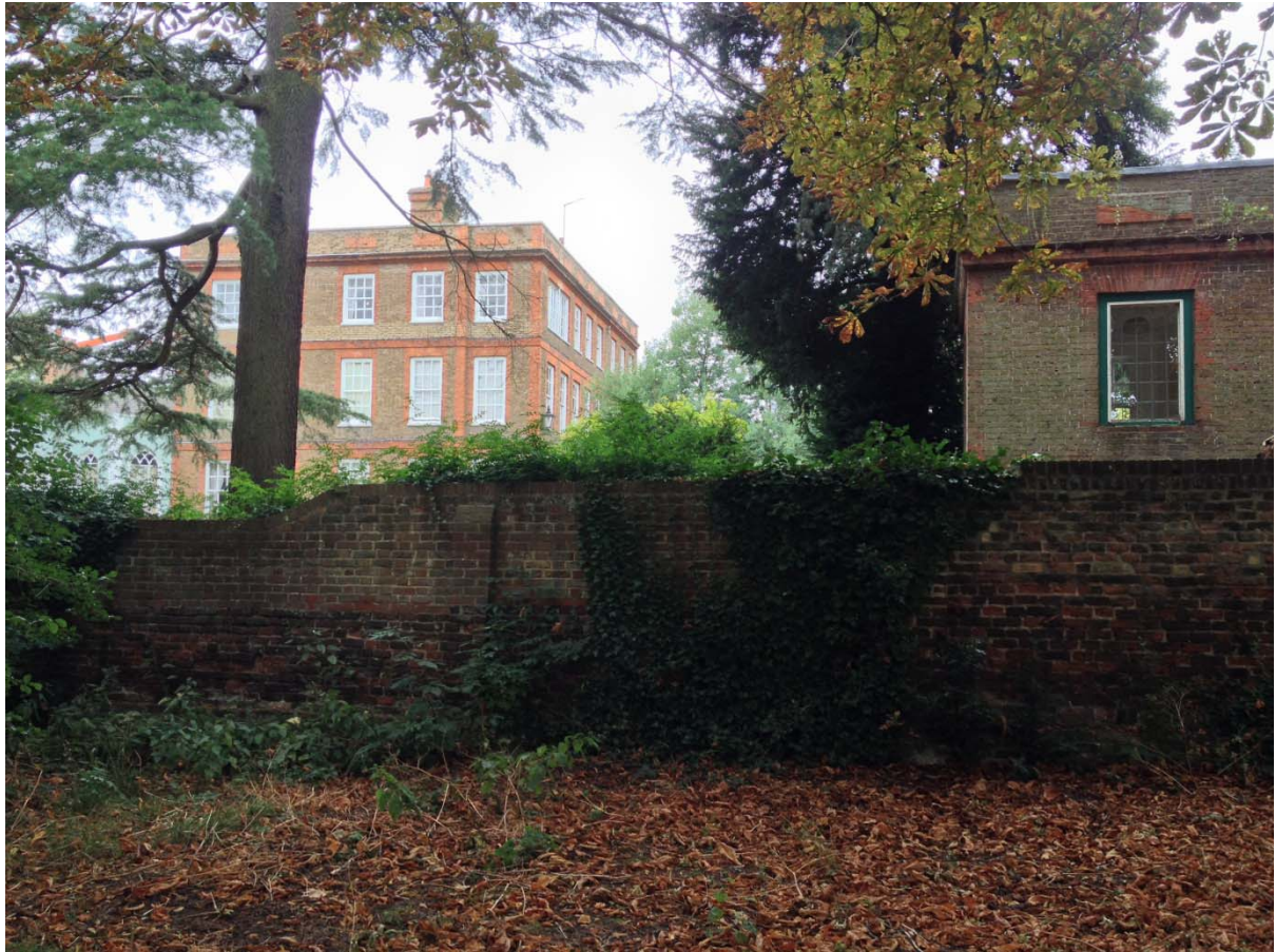
Fig.4 View of the Gazebo from Marble Hill Park to north-east.
