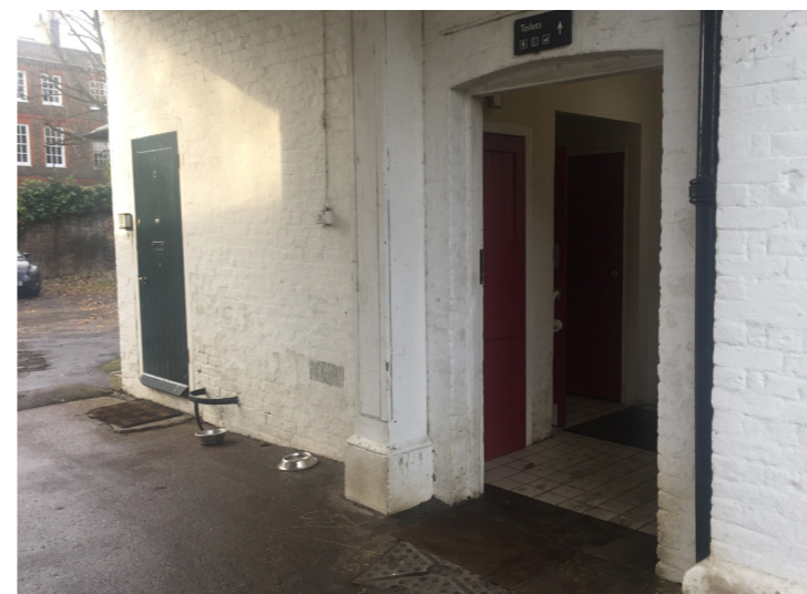
Existing door amended to create new entrance to overflow seating
