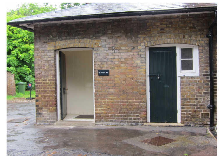
Existing Wc's to be upgraded
