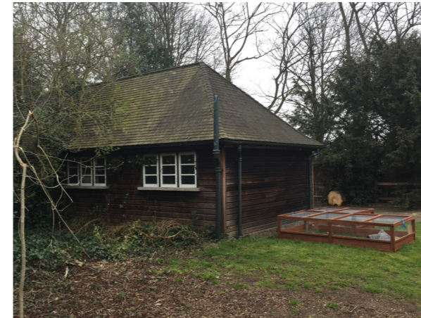
Former Changing Block, Scout Hall
