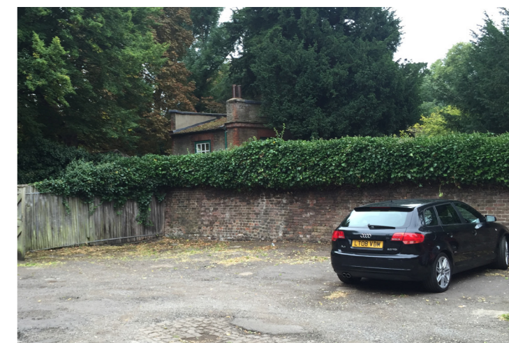
View of Boundary wall to Southend House from yard
