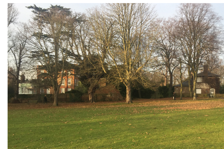
View of Southend House Boundary wall and Stable Block
