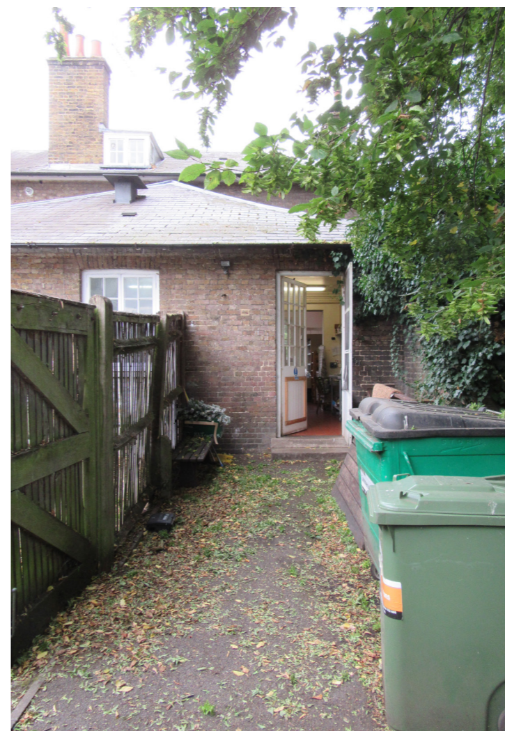
Existing bin store and kitchen door
