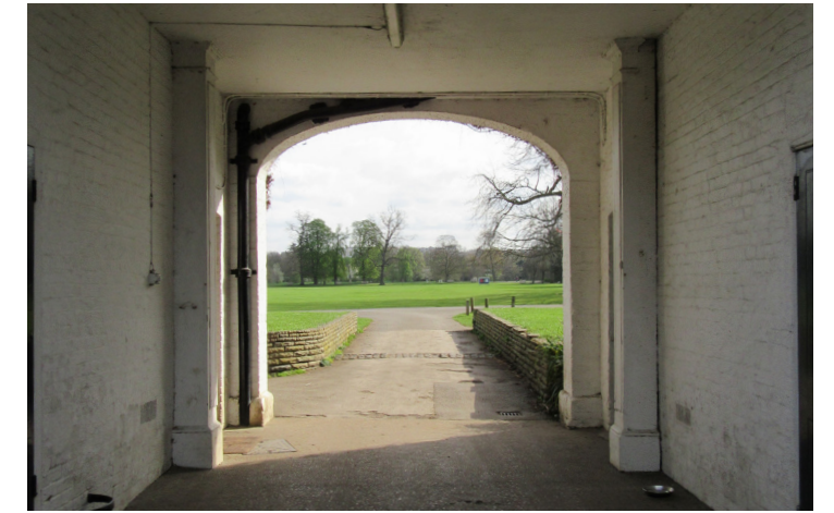
7. View from Stable Block to Great Lawn
