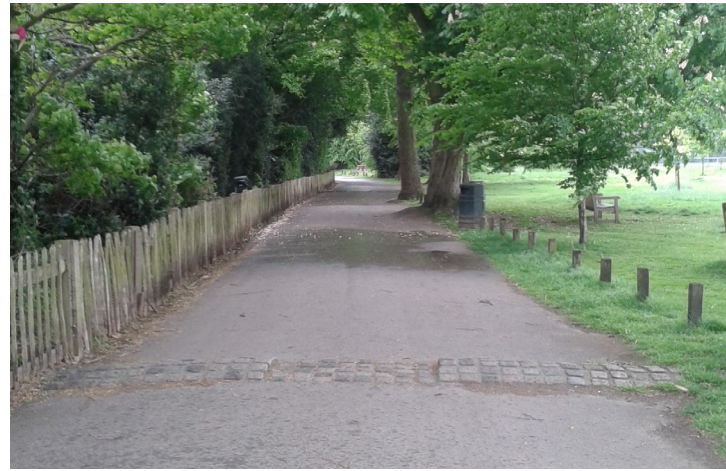
1. Delivery road from Richmond Road, looking north from Stable Block
