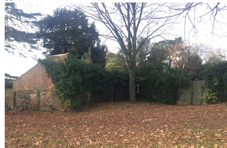
6. South End House boundary wall and gazebo with existing Stable Block fence
