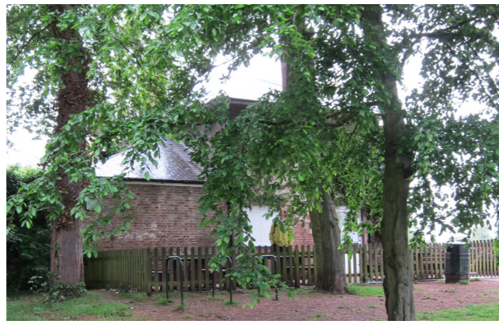
6. South elevation, boundary wall to yard. Ground falls away towards western meadow
