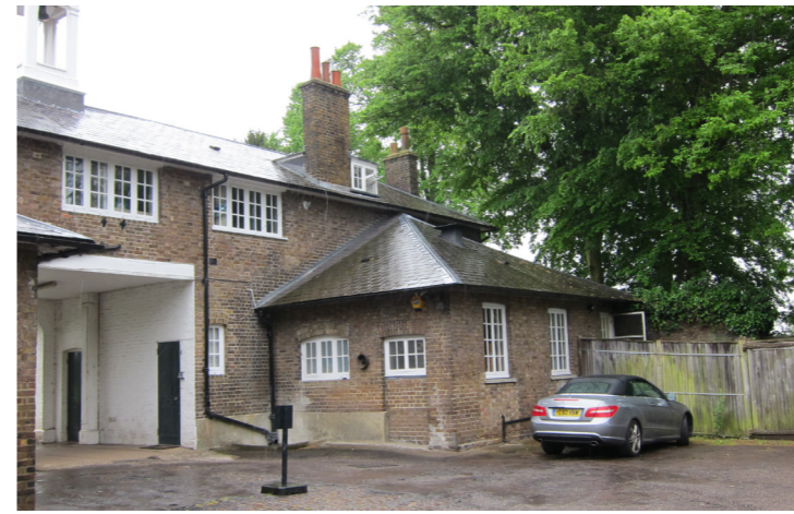
9. West (rear) elevation from yard
