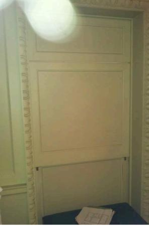
A typical 'sliding sash shutter' these are found on the second floor and are formed from two vertically sliding shutters, one going up, the other down. Both are fitted and equipped like a conventional sash window would be with weights, cord and a pulley.
