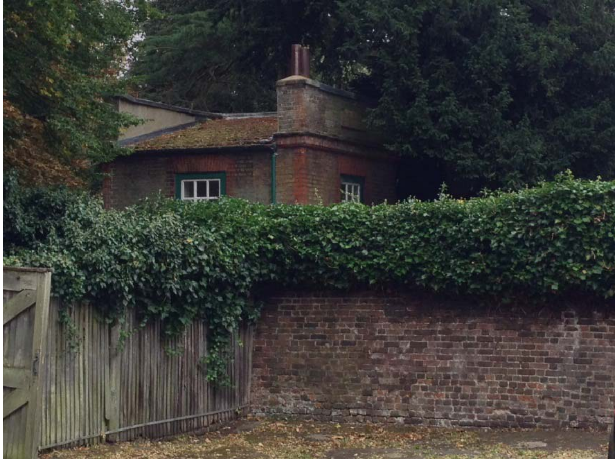
Fig. 3 View of the gazebo from Marble Hill stable block yard.
