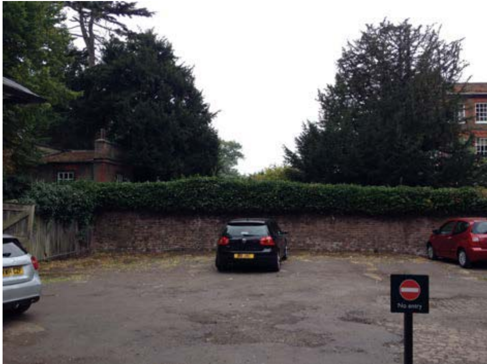
Fig.5 Western boundary wall
