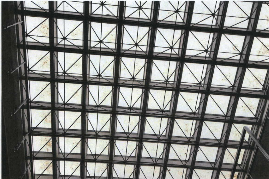
Internal view of Coxdomes and spaceframe
