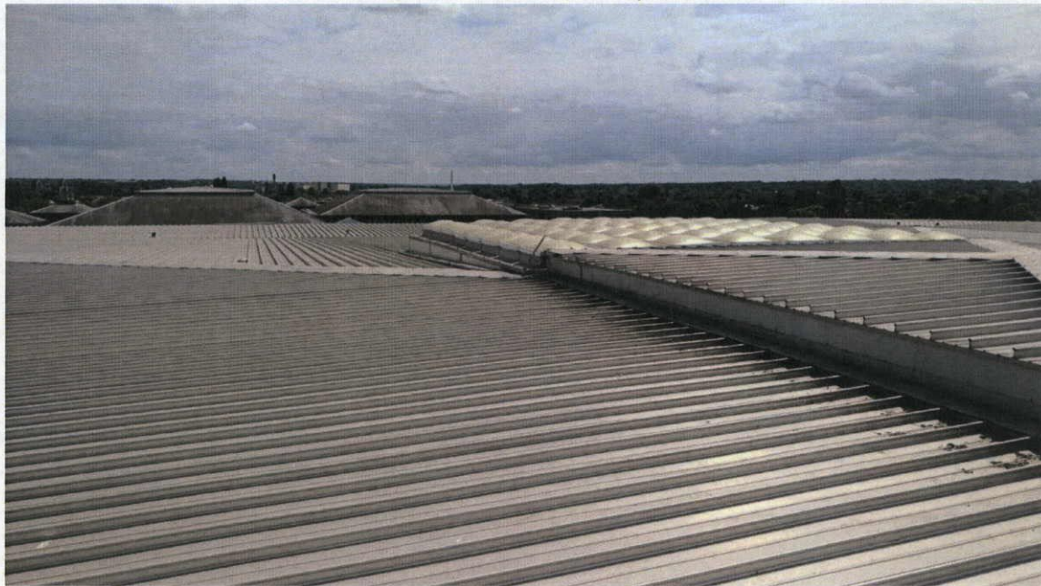
External view of Coxdomes and Kalzip roofing
