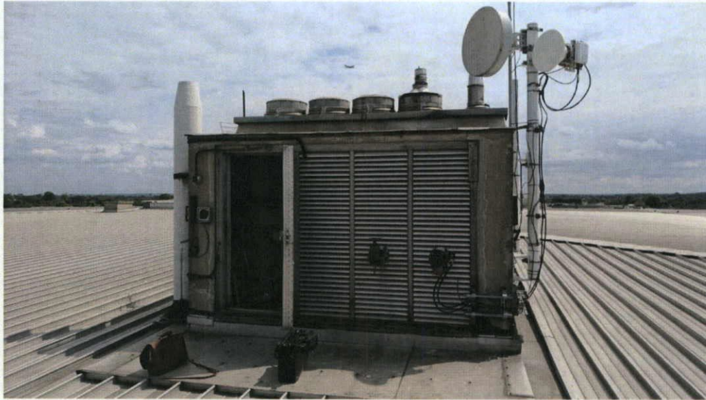
Existing structure with roof access ladder within
