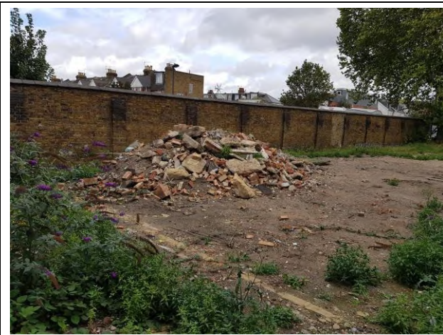
Fleming Dining Area demolished in north of site.
