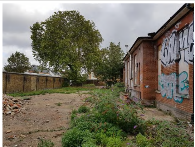
Northern edge of Fleming Lodge , boarded up and no longer in use.
