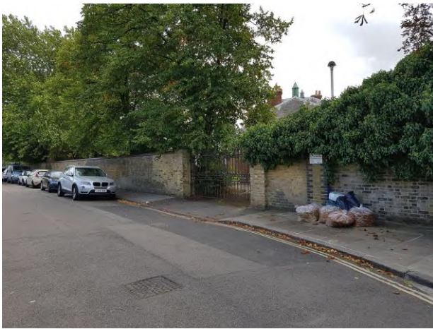
Northwest entrance to the site, no longer in use.
