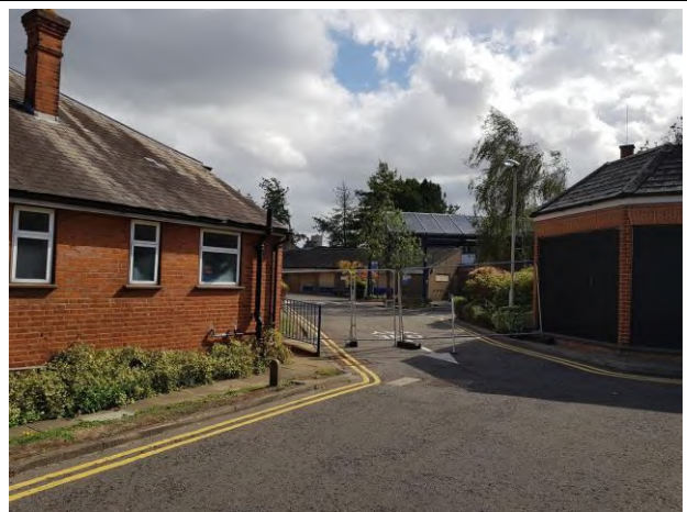
Looking southeast from parking area. Beatrice Lodge still in use as offices (left). Other buildings are fenced off and boarded up.
