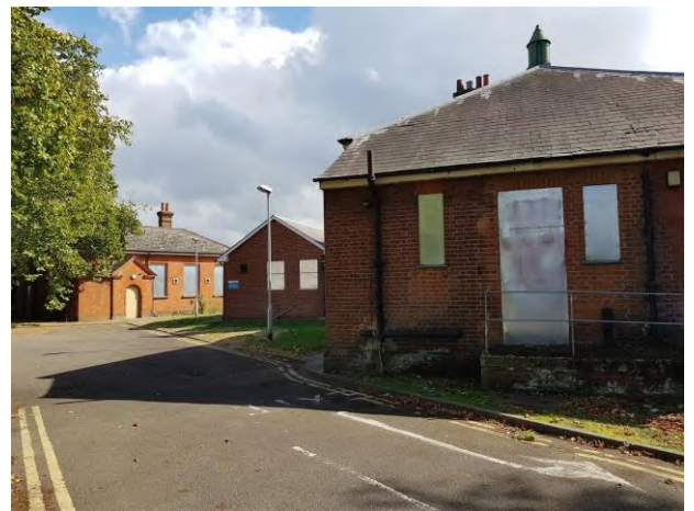
Looking east from northwest entrance to site at Workshop and Recreation Hall (left) and Elizabeth Lodge (right).
