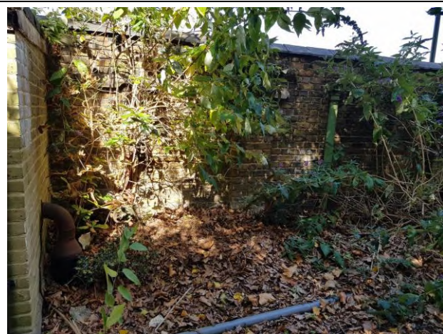
Possible tank base adjacent to gas cupboard.
