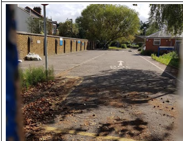
Looking south down the eastern boundary of the site at bungalow ward buildings.
