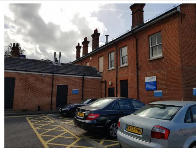
Looking southwest from parking area at one of the main hospital buildings, boarded up and no longer in use.
