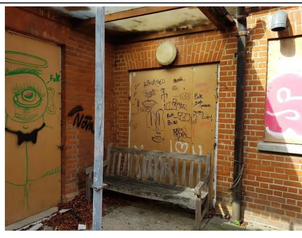
Plant room door on the ground floor of the Laundry House.
