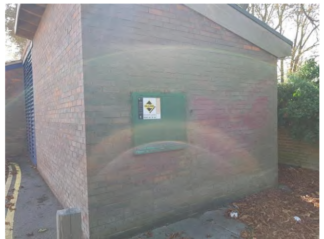
Location of diesel fuel tank and generator, in the northwest of site.
