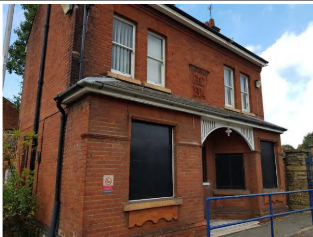
Victorian Doctors Residence building, west of the site entrance.
