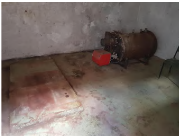
Disused basement plant room beneath Fleming Lodge , with tank base.
