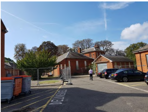
Looking west from parking area at Elizabeth Lodge . Waste storage (bins) located on the left.
