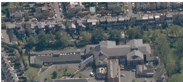
Figure 11: 77 – 93 Grosvenor Avenue street façade and birds eye view of rear elevations.
