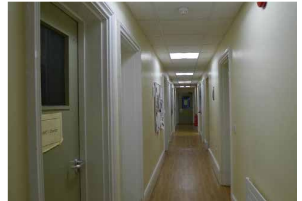
Figure 4.10 Interior of the Administration Building, showing modern suspended ceilings, fittings and fixtures associated with its current office use.
