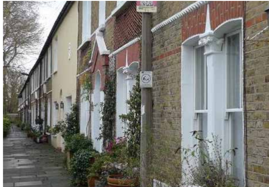
Figure 5.12 Nos. 1-13 Lodge Avenue.
