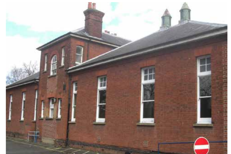
Figure 4.5 The west elevation of Elizabeth Lodge (1903-4).
