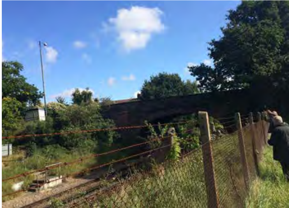
3 / Road bridge over railway line to north
