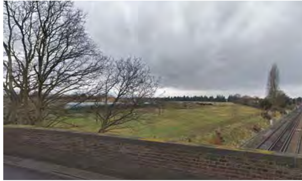
Existing View from Hospital Bridge Road
