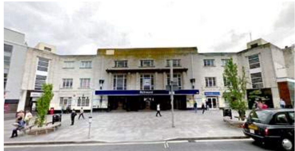
Richmond Station, Richmond
