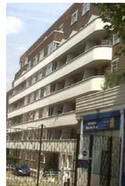
Horizontal band found on Art-deco building; Lichfield Court
