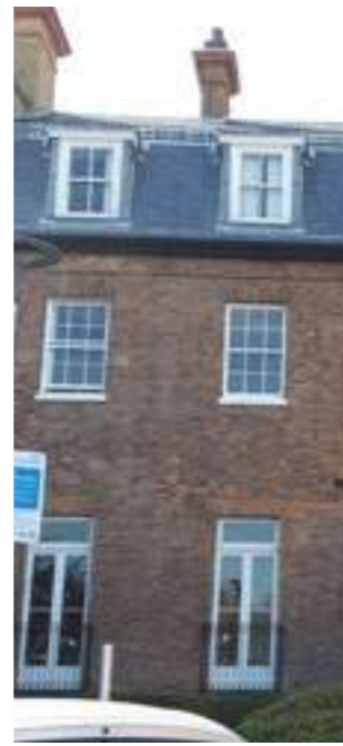
Existing window & balustrade in Listed Building
