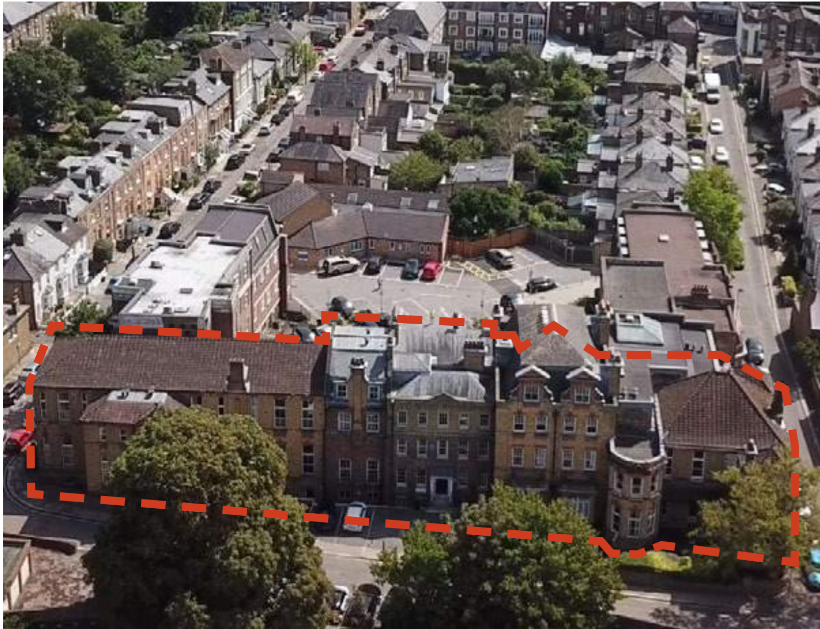
Aerial View of Richmond Royal Hospital West
