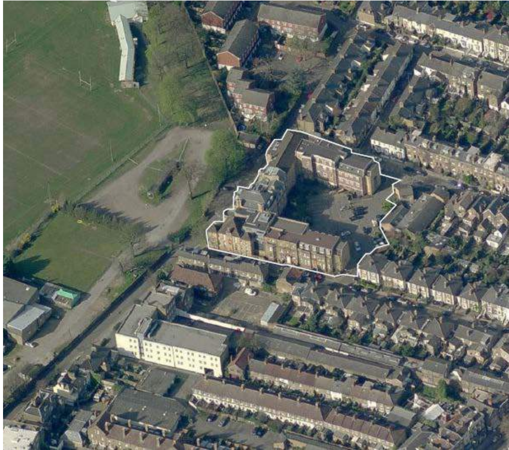
Figure 2: The Site – aerial view (Source: Google Maps)
