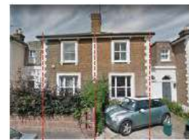
Typical Houses along Shaftesbury Road
