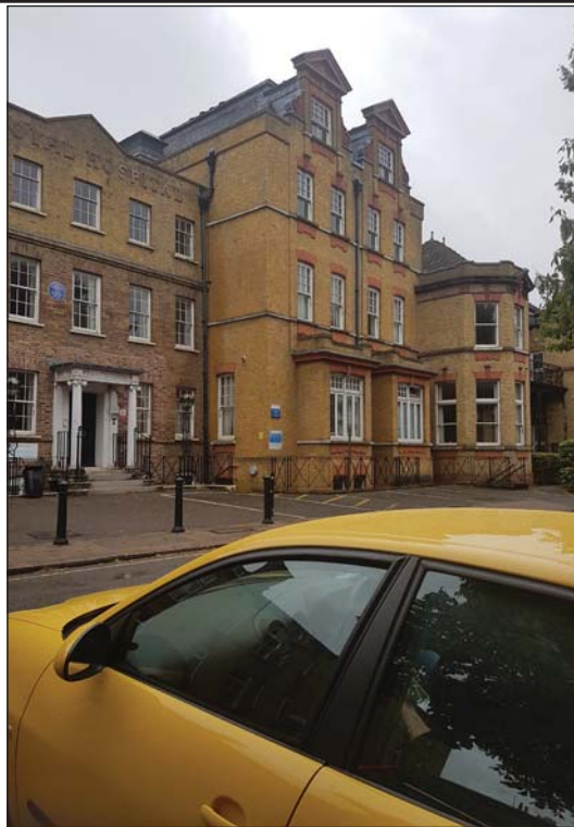
Plate 3. Site looking south-east from west.
