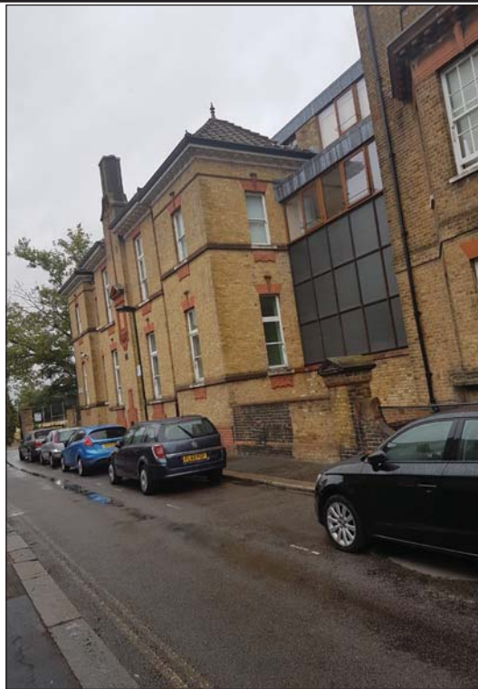
Plate 5. Site looking west from south.
