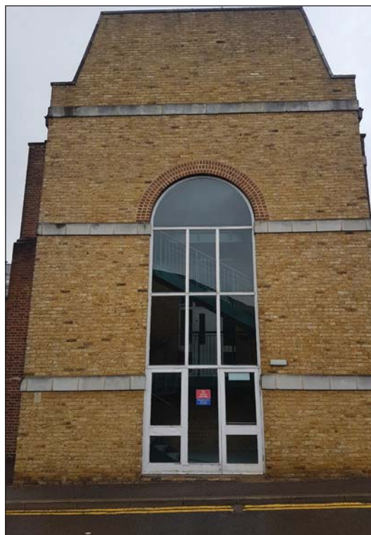
Plate 10. Site looking west from east.
