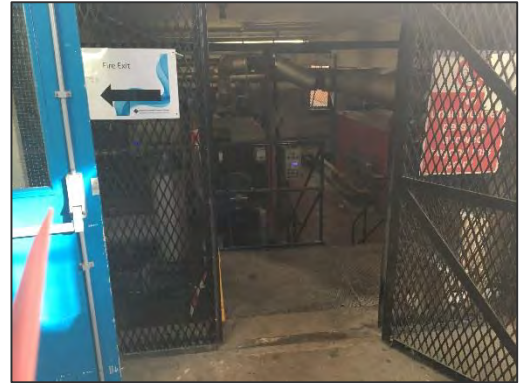
Photograph 4: Facing into Plant Room.
