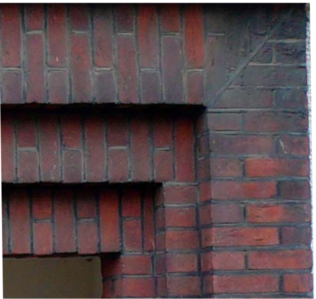
Brick work details and corbelling features. - Modern example above
