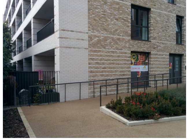
Brick colour/type change in courtyards - Barrier Park
