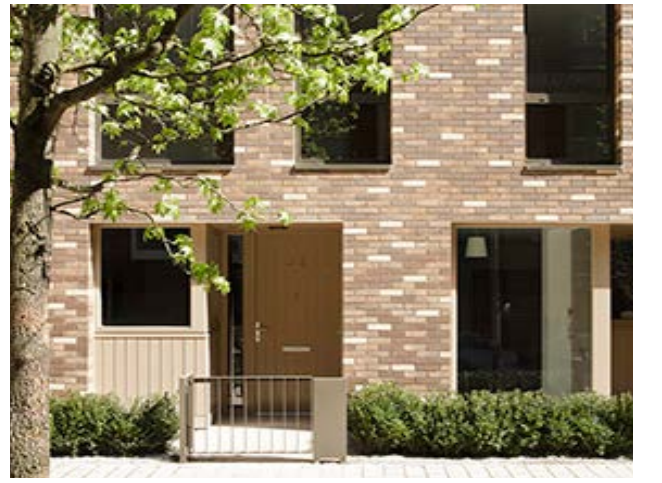
Inset entrances - St Andrews Maccreanor Lavington Architects
