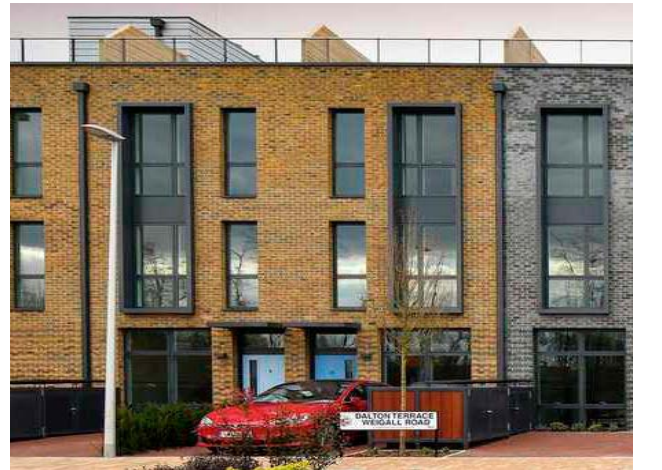
Kidbrook Houses - Paired entrances with flat roofs
