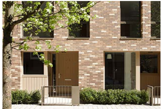
Inset entrances - St Andrews Maccreanor Lavington Architects
