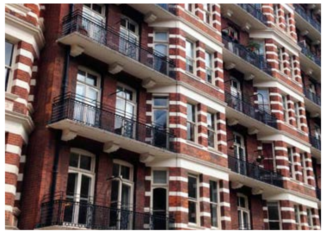
Wrapping balcony forms in mansion blocks
