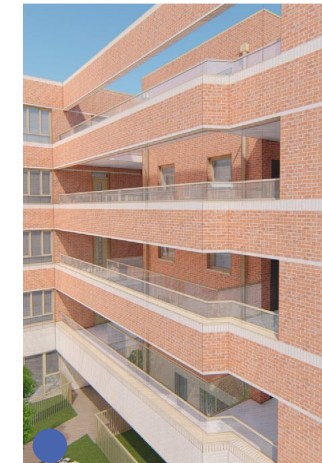
Balcony type 03 Deck Access Elements - Brick work with glass and metal railing
