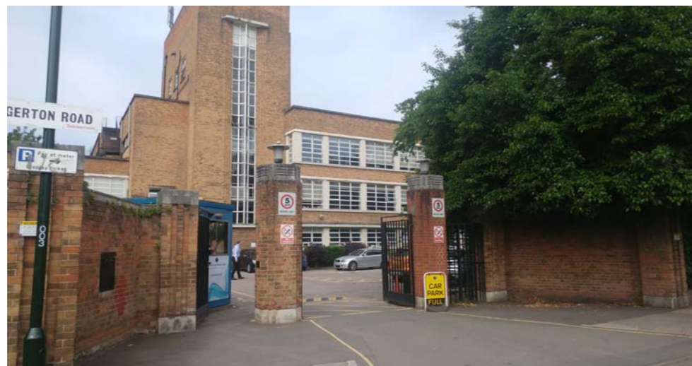
Existing brick entrance piers to be retained and incorporated into proposed boundary treatment along Egerton Road
