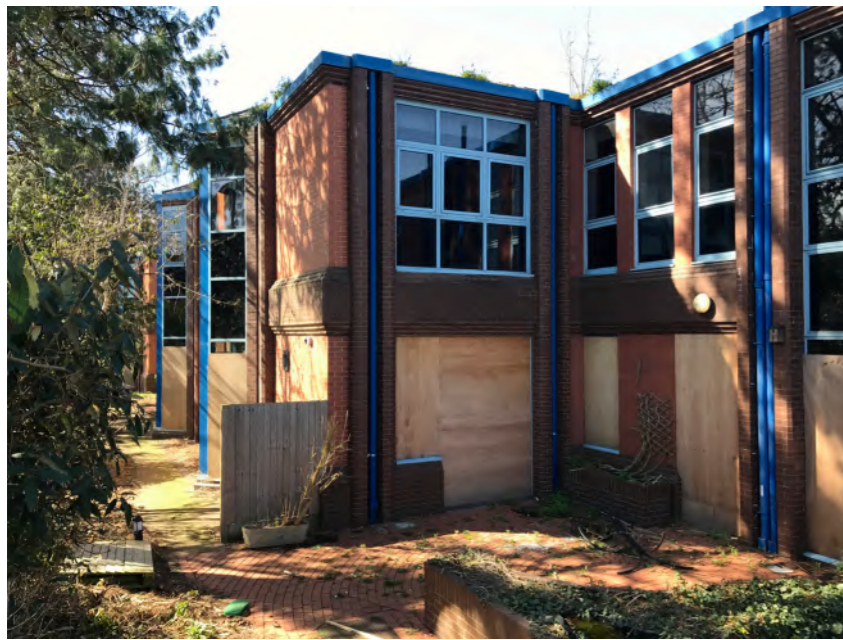
Building in the south-west corner of the site
