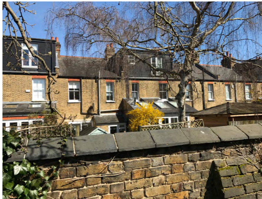
View of houses fronting Grosvenor Avenue
