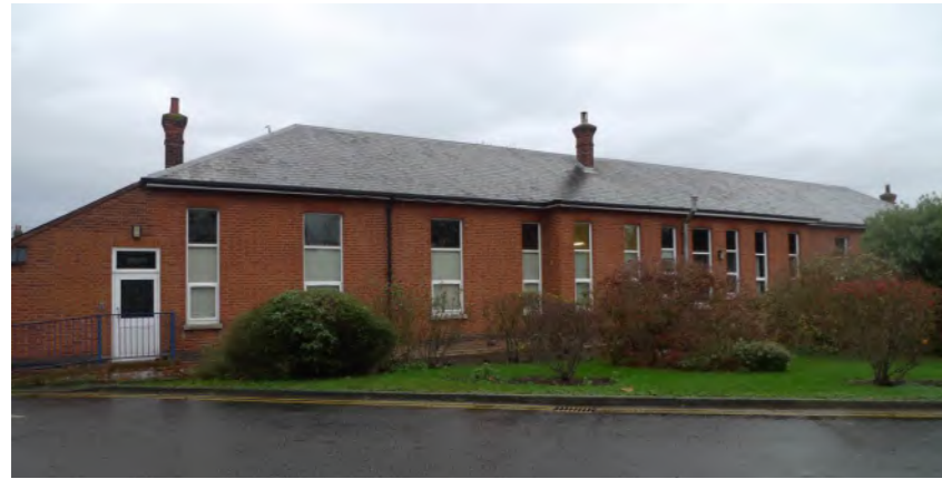
Southern elevation of Beatrice Ward, constructed in the 1920
