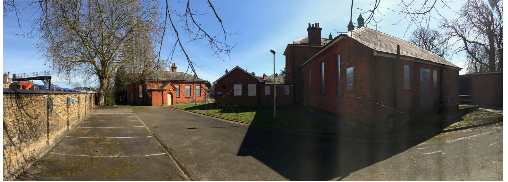
Panorama of buildings on site, south-east
