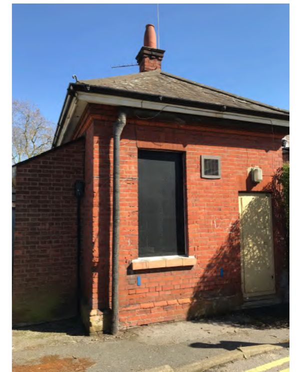
The Gatehouse [C]
