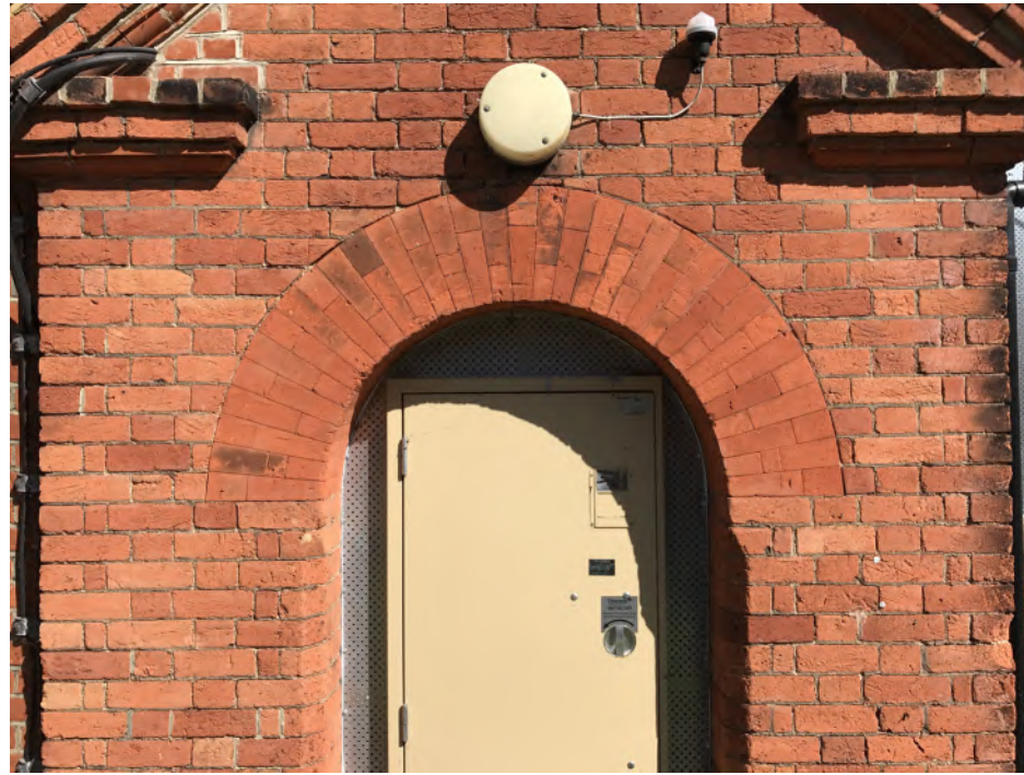
Gauged Brickwork, on site
