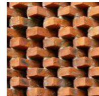
Red Gauged brickwork, found on the BTMs
