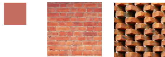
Gauged brickwork, found on the BTMs
