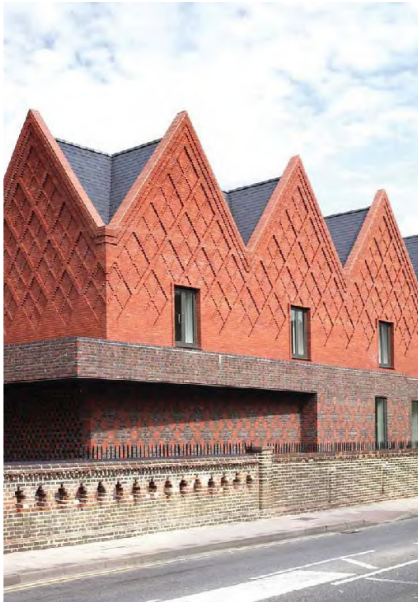
Example of contemporary detailing of vernacular form
