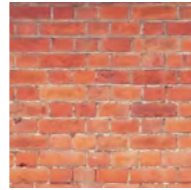
Red Gauged brickwork, found on the BTMs
