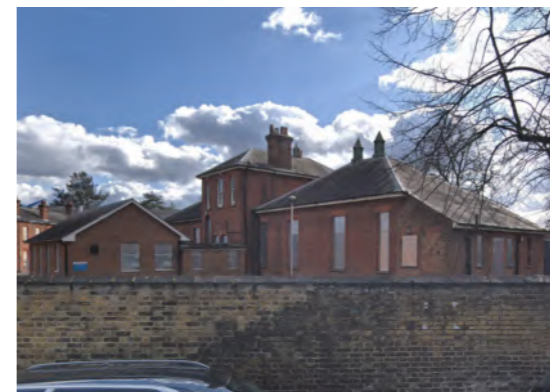
Elizabeth Lodge North Elevation
