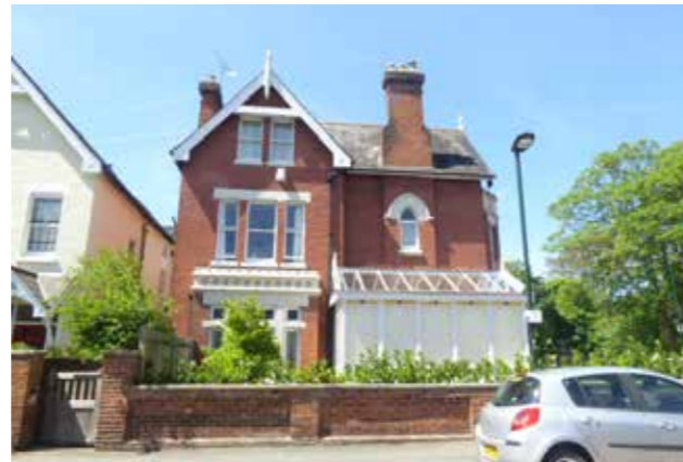
14 - Lower Teddington Road (upper west side)
