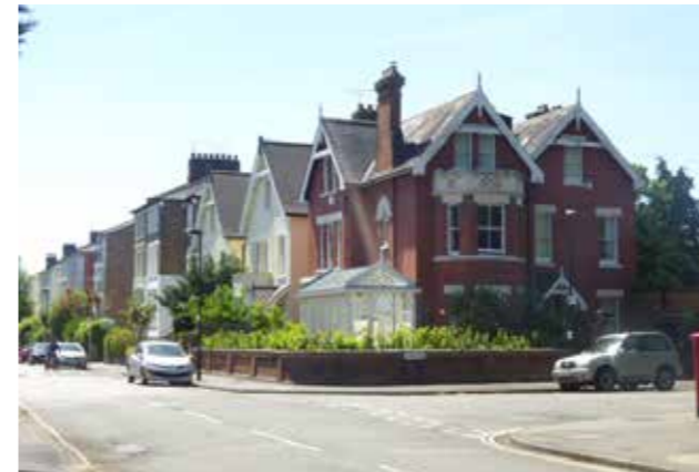
15 - Lower Teddington Road (upper west side)
