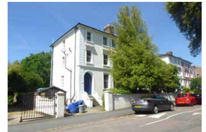
4 - Lower Teddington Road (upper west side)
