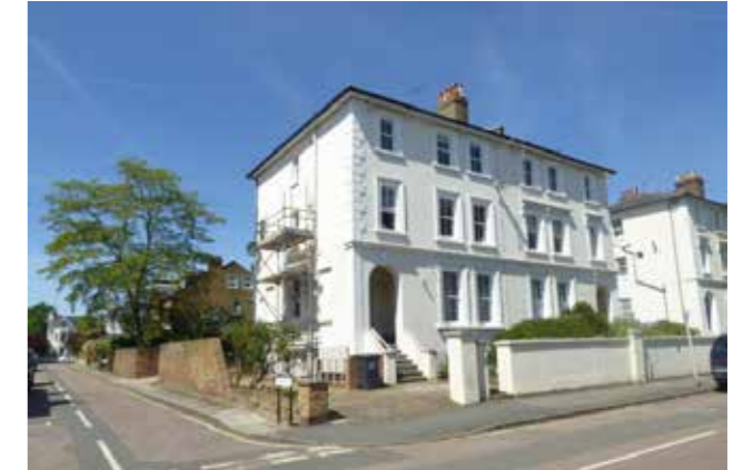
2 - Lower Teddington Road (upper west side)
