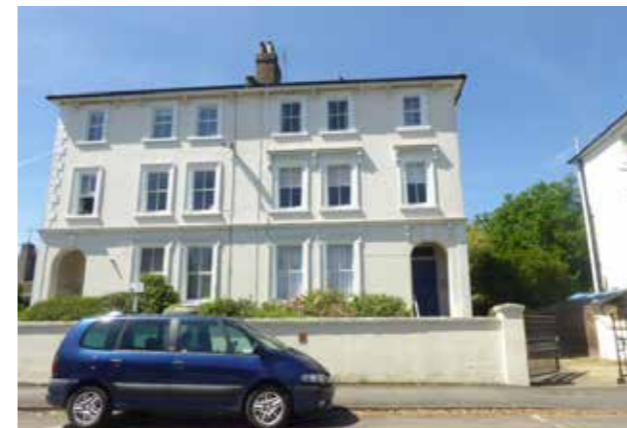
3 - Lower Teddington Road (upper west side)
