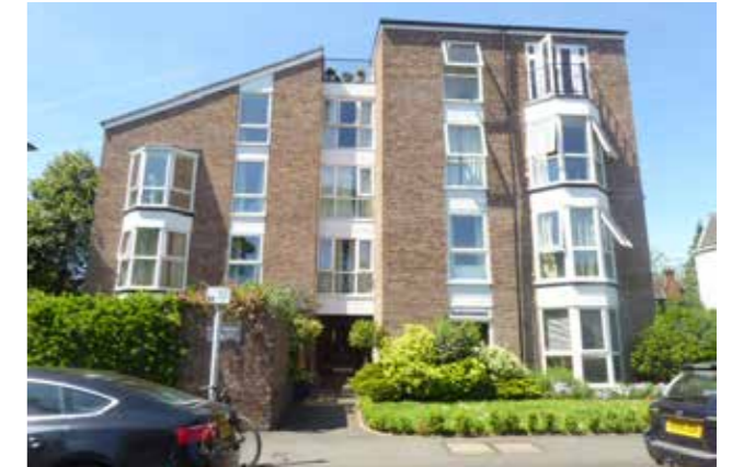
7 - Lower Teddington Road (upper west side) Winterton Court
