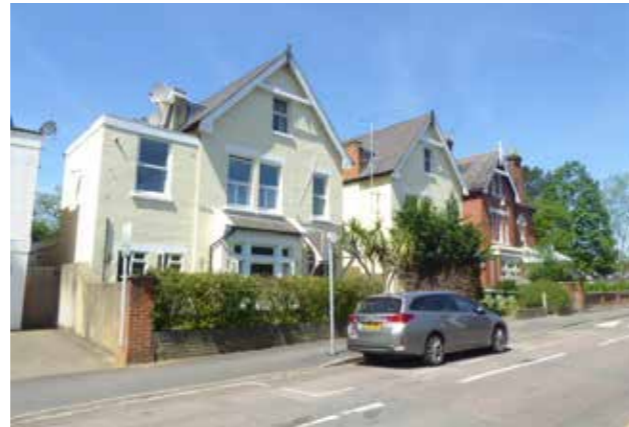
11 - Lower Teddington Road (upper west side)
