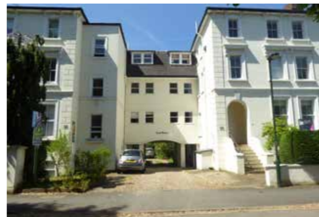
5 - Lower Teddington Road (upper west side)
