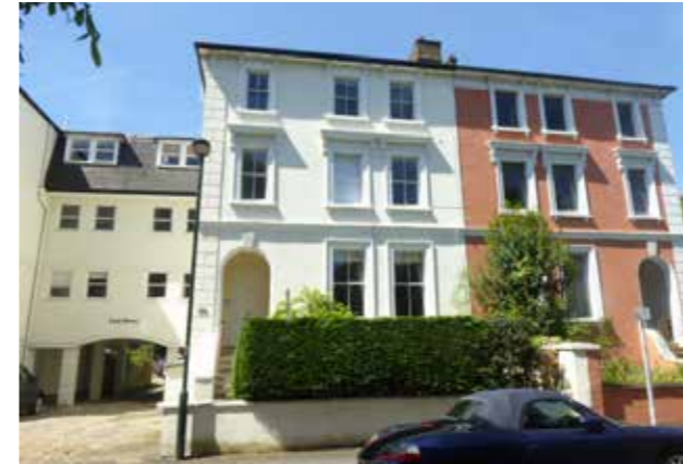
6 - Lower Teddington Road (upper west side)
