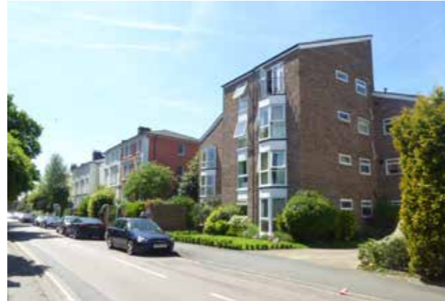
8 - Lower Teddington Road (upper west side)
