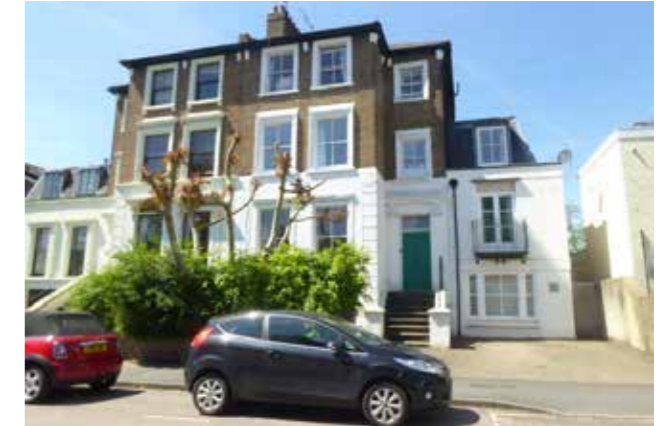
10 - Lower Teddington Road (upper west side)
