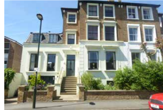
9 - Lower Teddington Road (upper west side)
