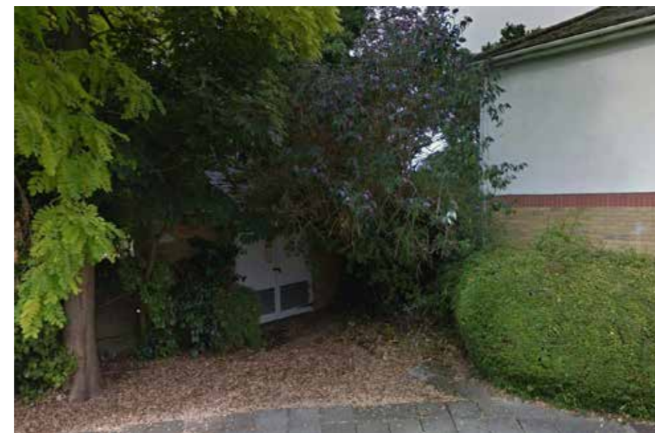
Above: General view of existing electrical sub-station access to the west of the application site (overgrown).
