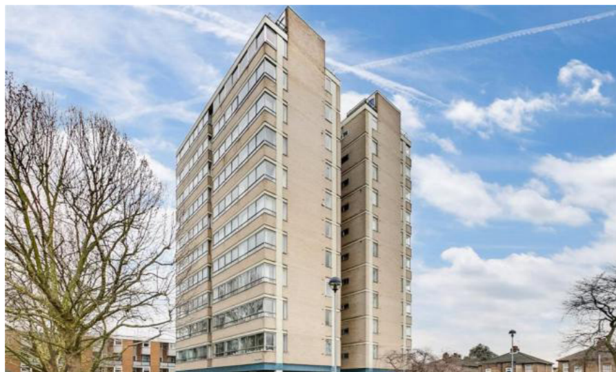
The Towers, 12 storeys
