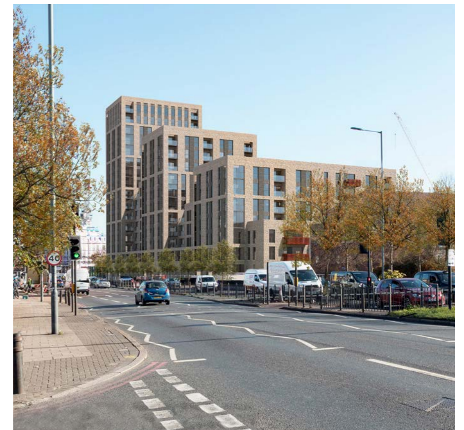
4 - Former Homebase site, Acton, Hammersmith and Fulham. Barratt London and TP Bennett
