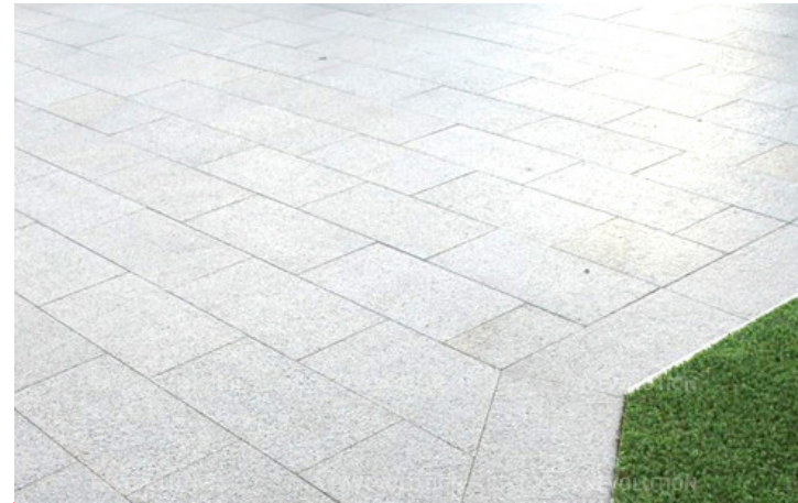
Granite paving with frame
