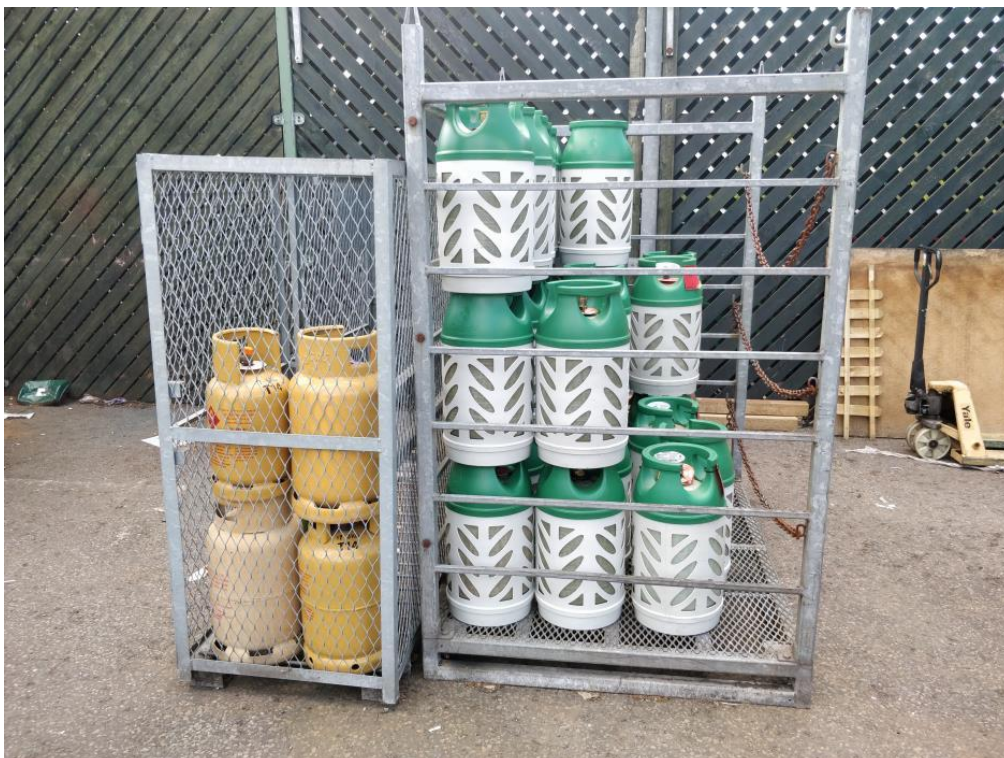
Photo 10: Gas canister storage in Homebase delivery yard
