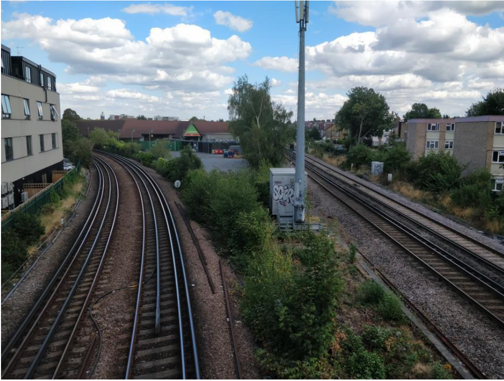
Photo 20: National Rail infrastructure
