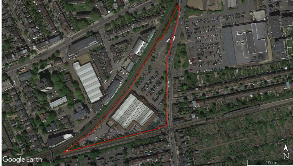
Figure 3.1. Aerial photography showing site boundary and surrounding landscape
