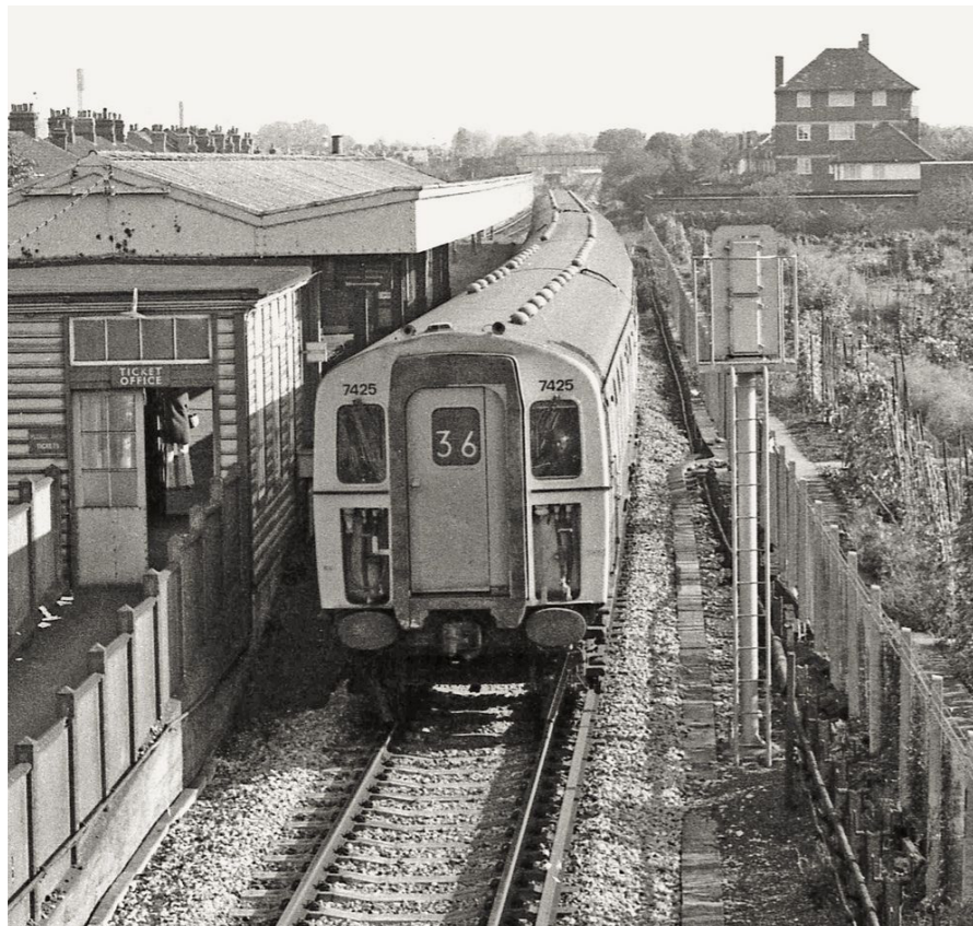
North Sheen station 1974
