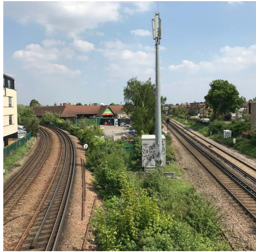
1. View looking east towards the site
