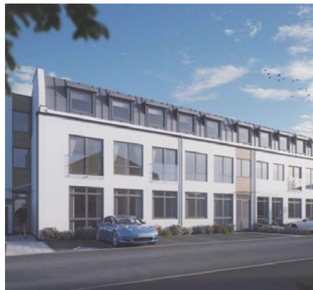
C - Manor House, Bardolph Road
