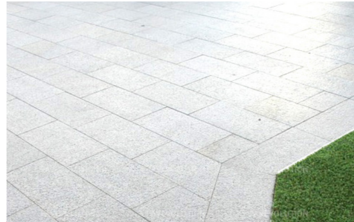
Granite paving with frame
