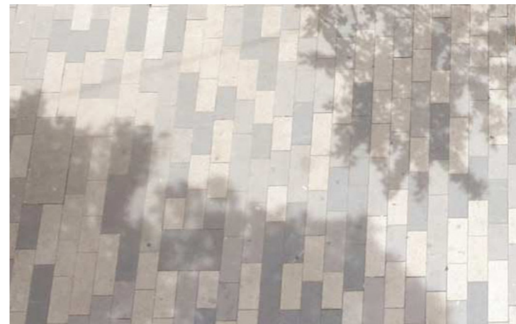
Granite setts (Coloured mix)
