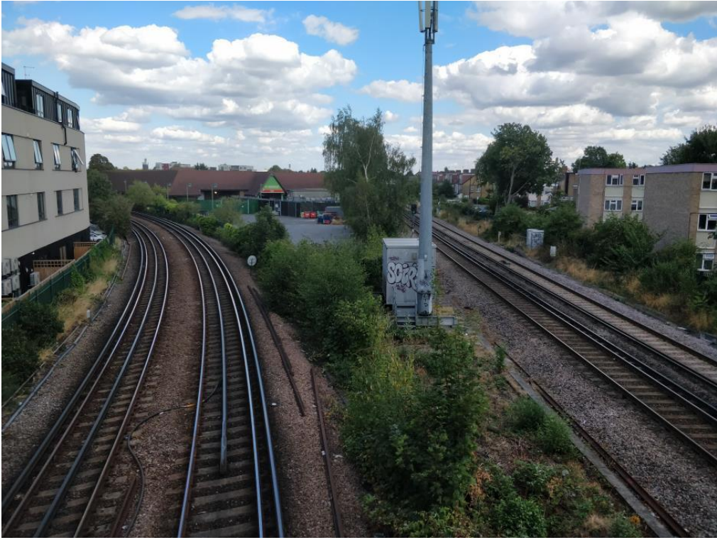
Photo 20: National Rail infrastructure
