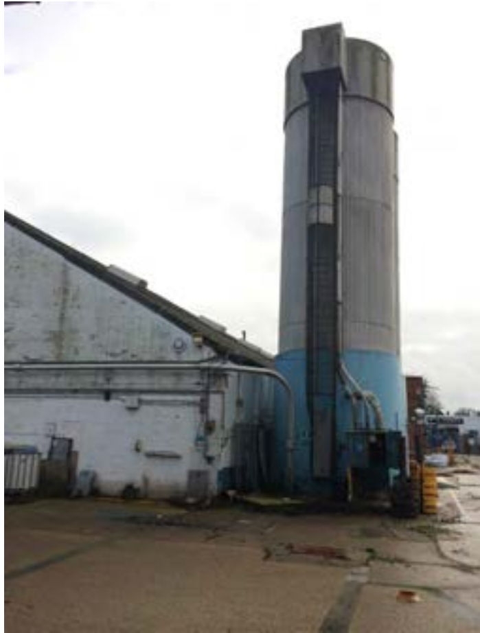
Plate 13: Northern flour Silo viewed from the North.
