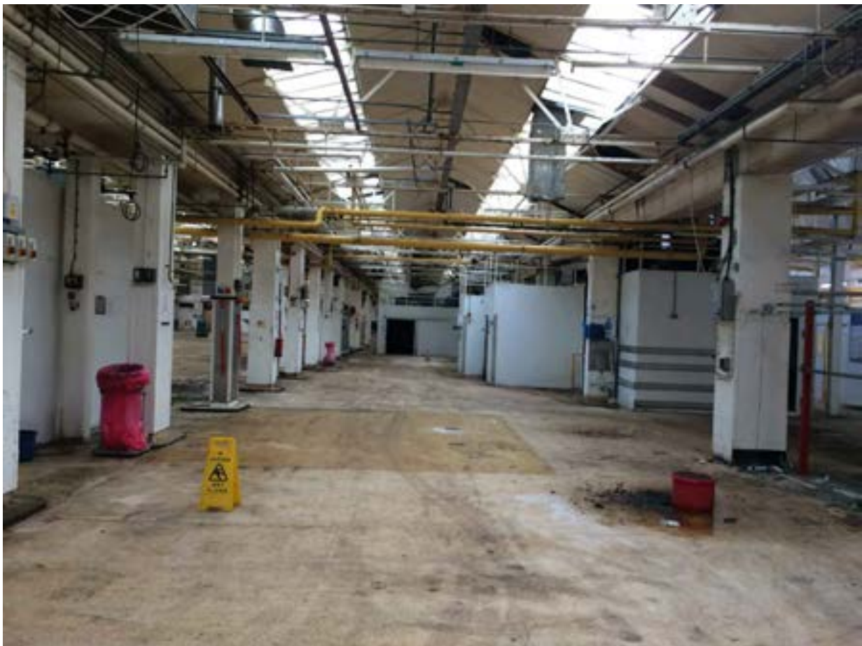
Plate 6: Main processing plant western half viewed North to South.
