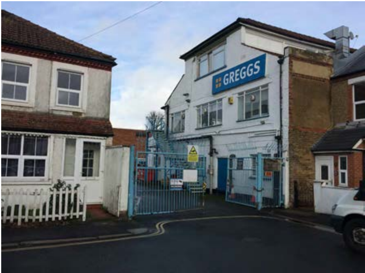
Plate 3: Gould Road administration block viewed from south-west.
