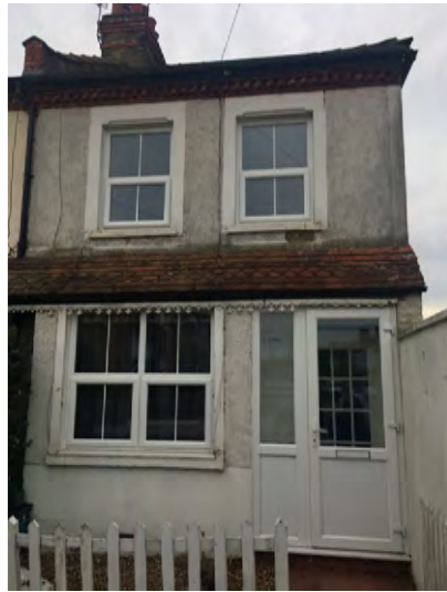
Existing house - No. 1 Gould Road
