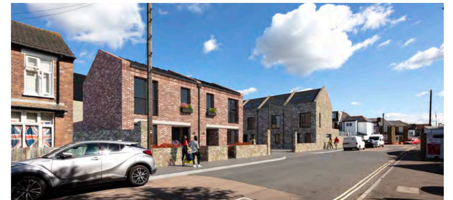
Fig 1 - Proposal adjusted to introduce the gable end condition that's typical to Edwin Road and signifies a turn (August 2018)
