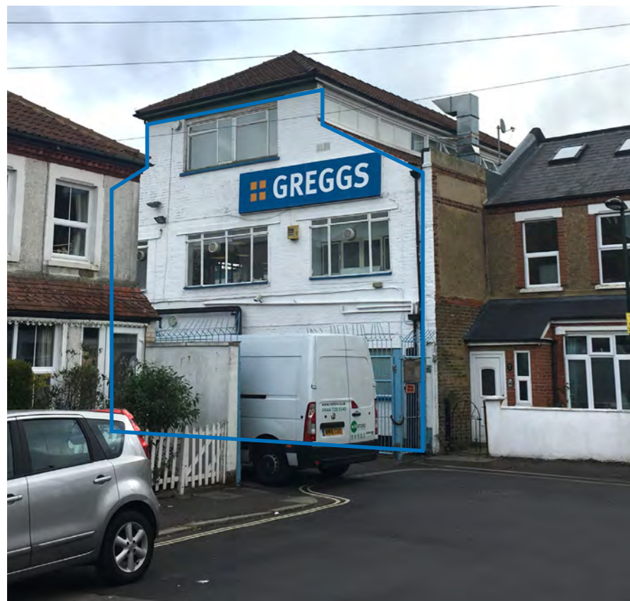
Site photograph showing lantern roof of existing Greggs building
