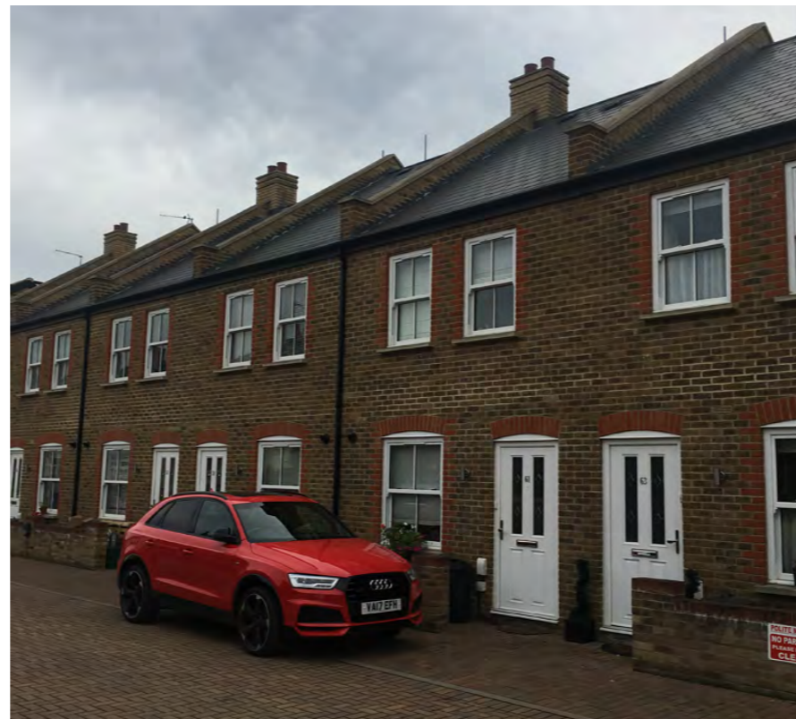
Photos of Norcutt House and terrace houses
