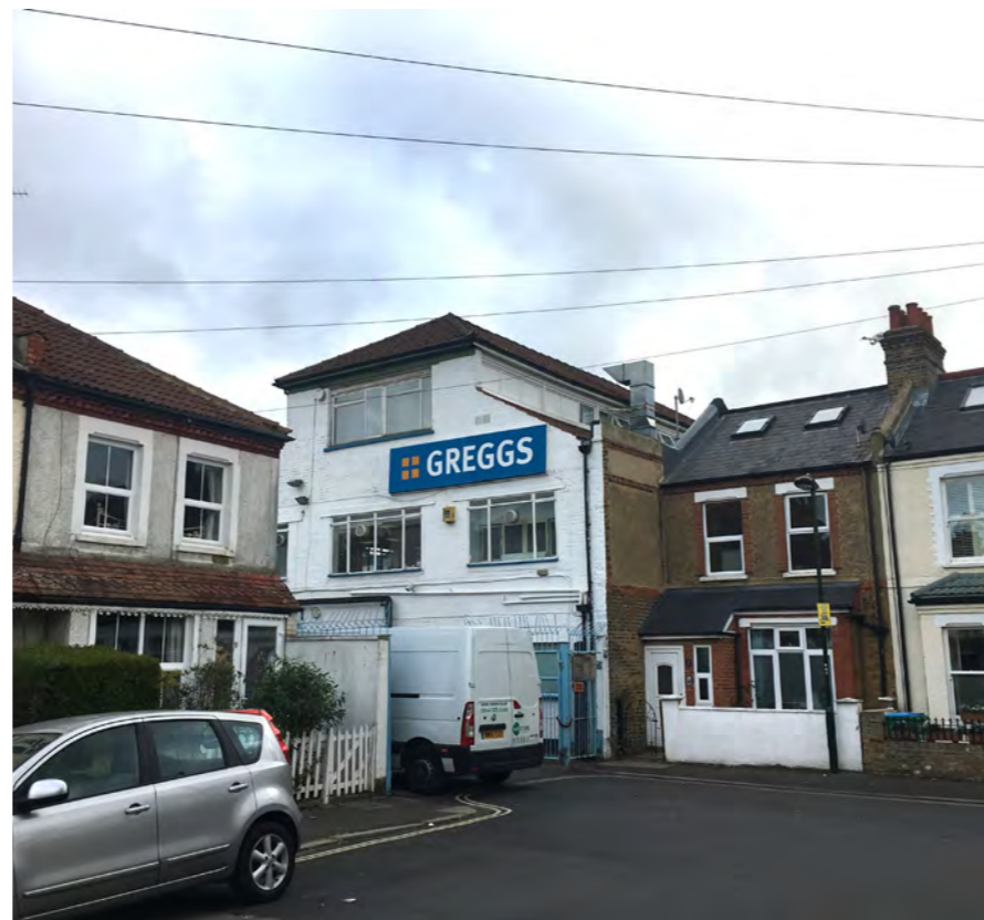
2. View looking towards Gould Road entrance
