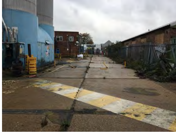
Photo 1: Overview of the southern section of the Site
